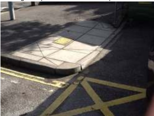
Drop kerb from disabled car parking space with no tactile pavers.
